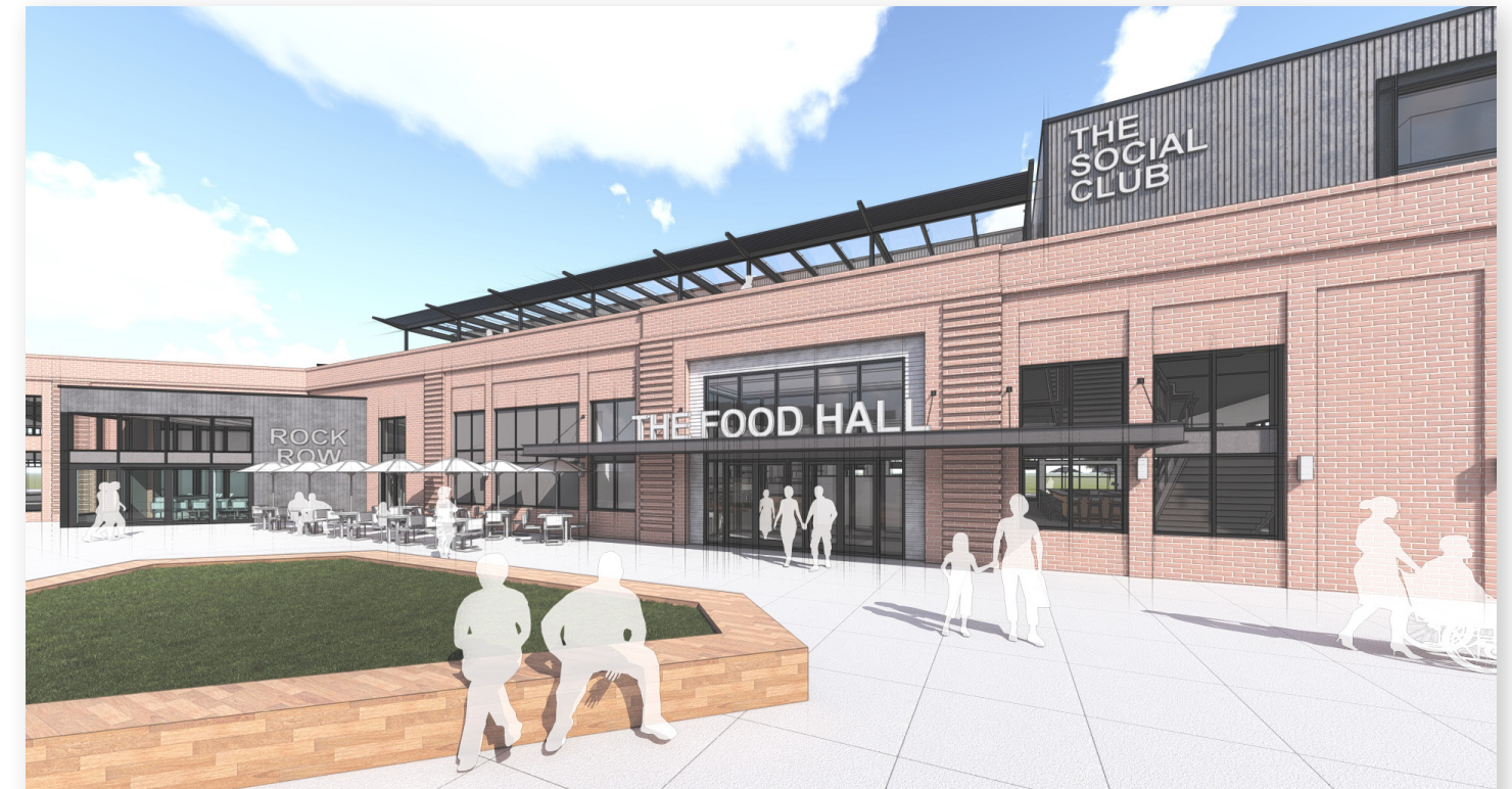
The centerpiece of a $2B, 100-acre mixed-use project in the Portland, Maine metro area, acclaimed New York chef Akhtar Nawab will be delivering his latest food hall project, Rock Row, later this year. This Brewery and Food Hall is strategically placed alongside manmade water features that will host seasonal hockey tournaments, summer water shows and boating. It's design features a focus on food and family on its first floor and a second floor that celebrates Maine's vibrant craft brewing and distilling scene with tasting rooms, a live performance/video projection stage, an indoor/outdoor oyster bar and concert venue seating. © 2023 Eimer Design
