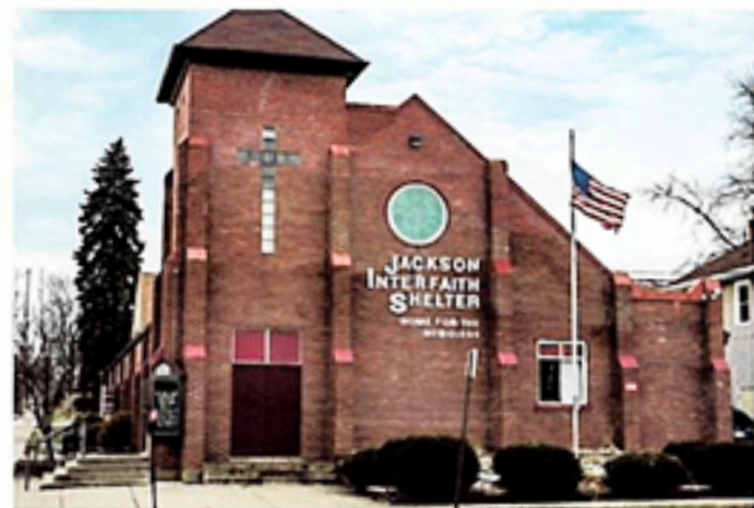
Shelter exterior before 2022 renovation
