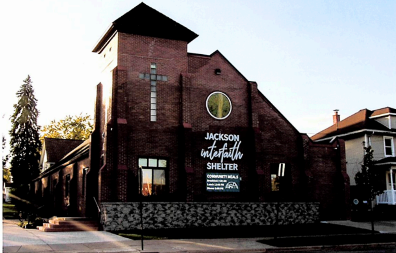
Shelter exterior after 2022 renovations
